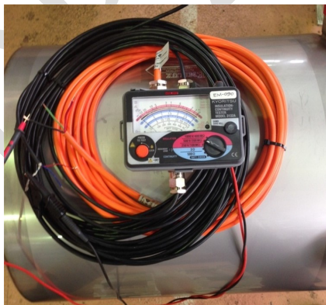
Figure 6: Megger testing from coil to earth in 500V range using approved equipment
