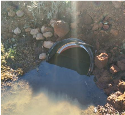
Pipe Insertion Installation
