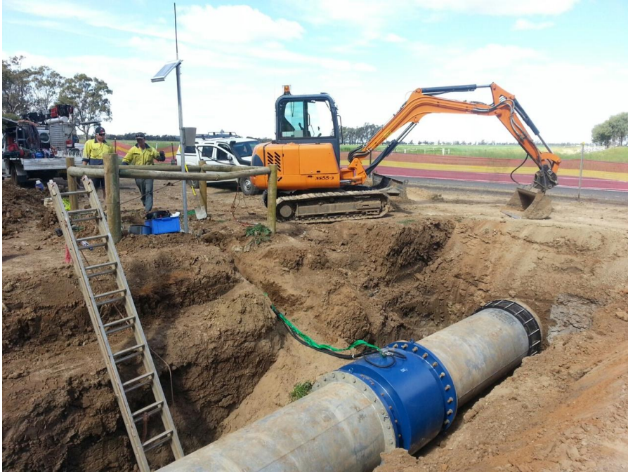
Mainline Pipe Installation
