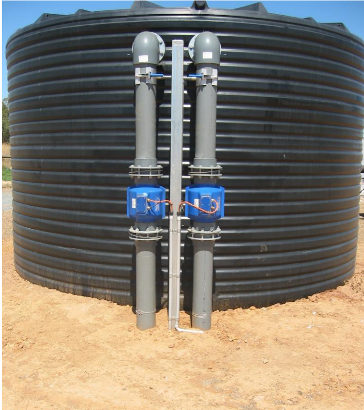
Vertical Tank Flanged Pipe Installation
