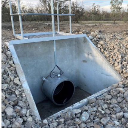
Pit Mount Installation (outside pipe)
