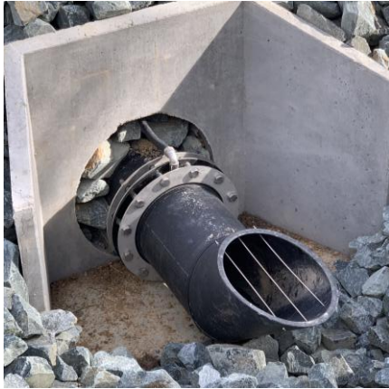
Pipe Insertion Installation
