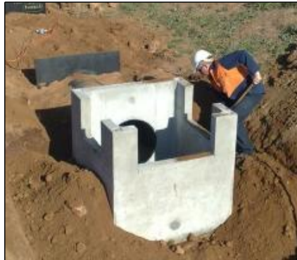
Pit Mounted Insertion Installation
