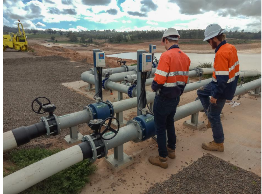
Tailings Dam Pipe Installation
